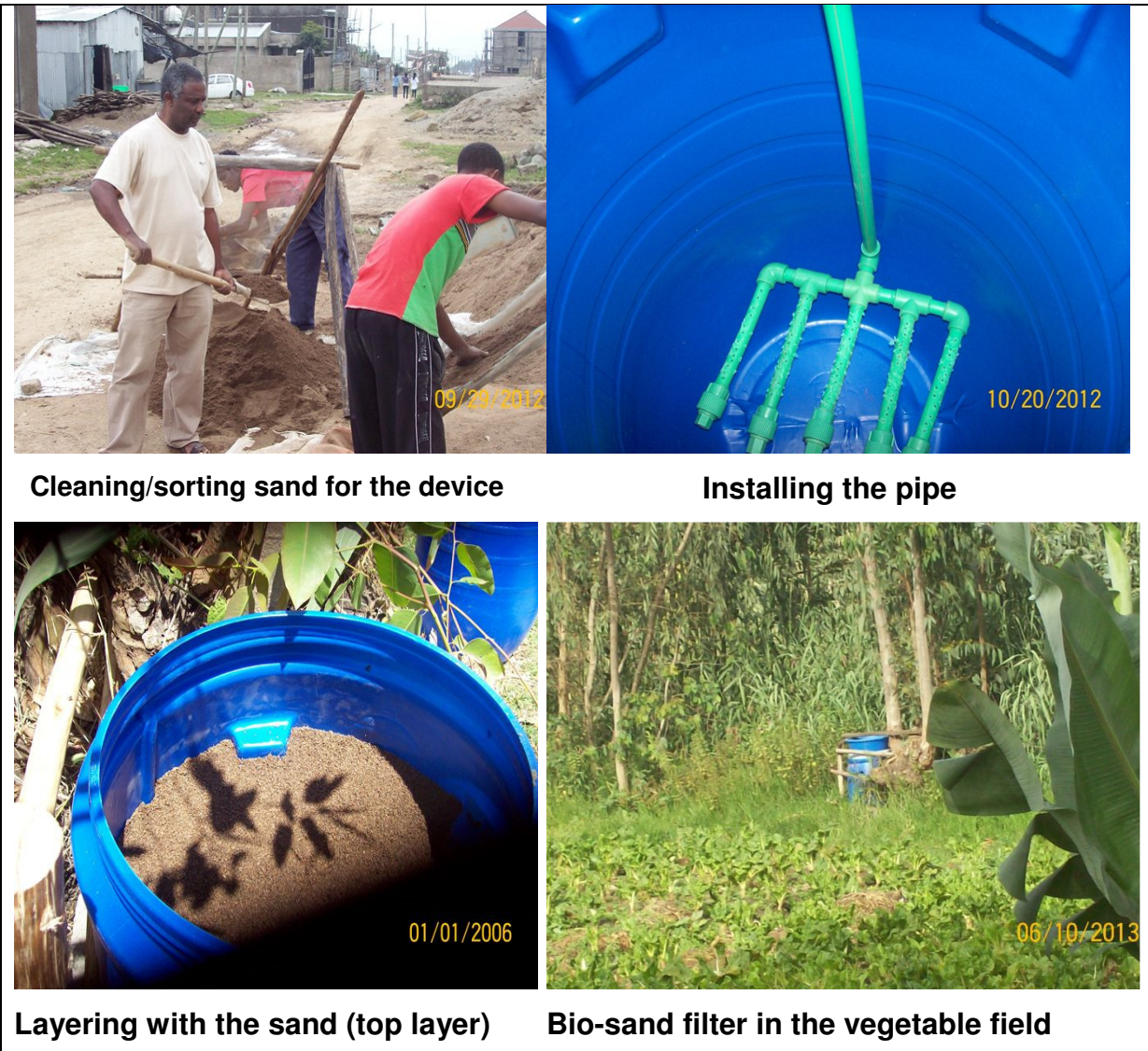
Figure 4.10: Process of bio-sand filter production, EcoHealth promotion, 2012 (Photograph by courtesy of EcoHealth promotion )
