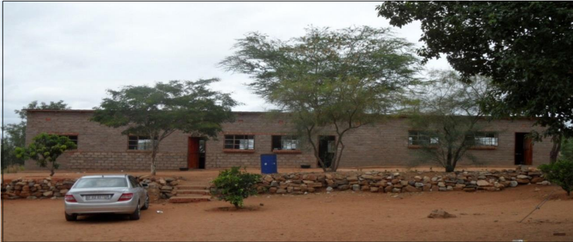
Figure 5.17: Shortage of classrooms leading to makeshift structures: Makushu Primary School Source: Photograph captured by the researcher in May 2011
