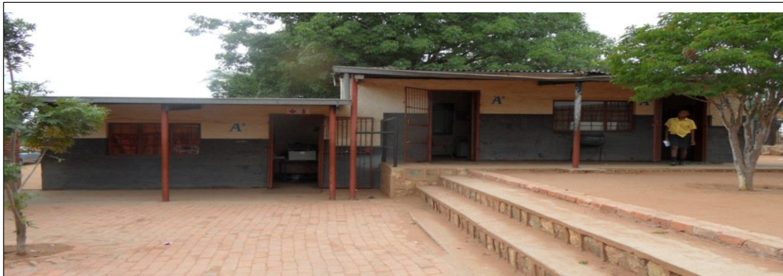
Figure 5.16: Administration building at Makushu Primary School in Musina Town Source: Photograph captured by the researcher in May 2011
