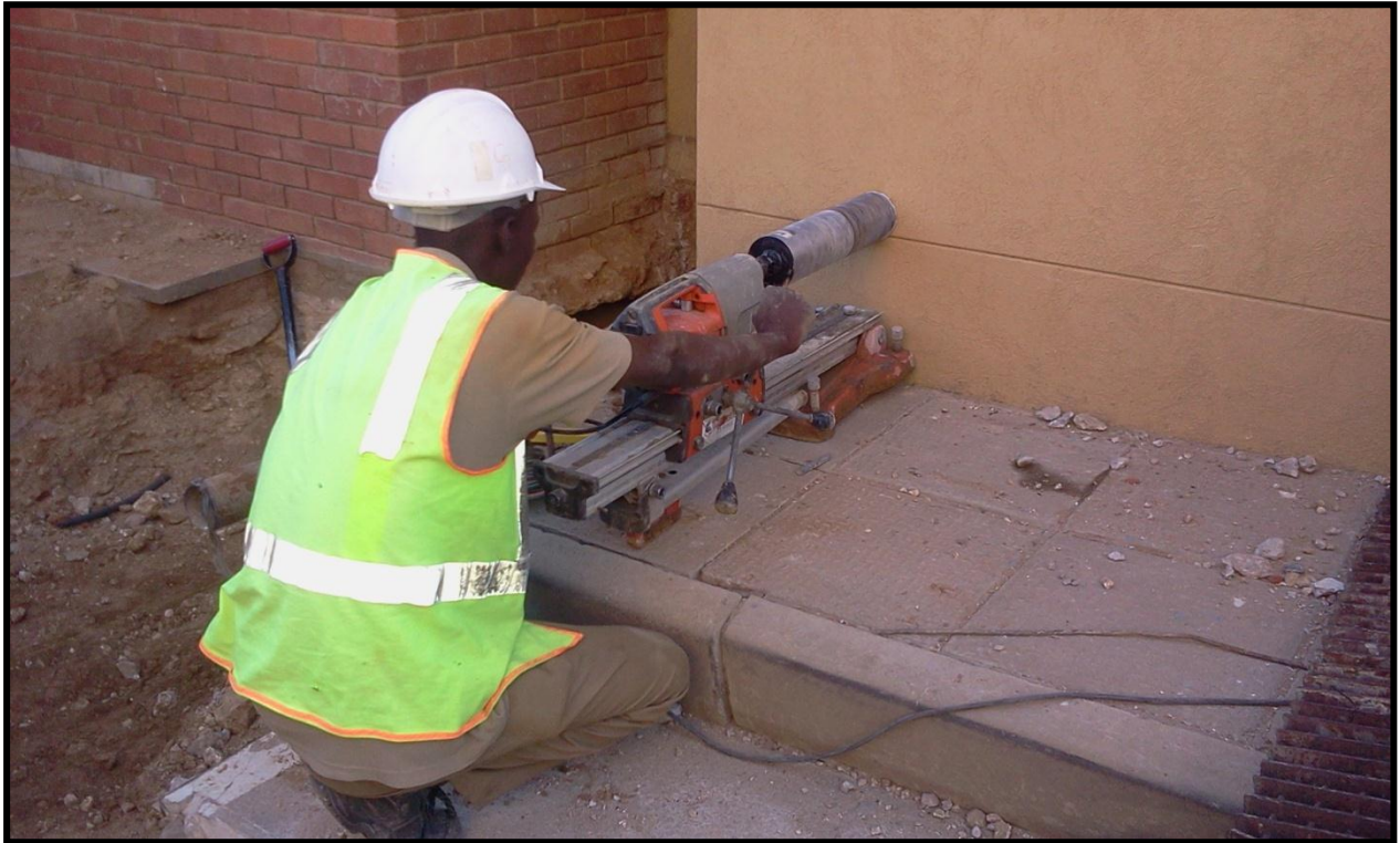
Figure 5.5 Picture depicting a worker exposed to vibration while adopting an awkward posture at the study site
