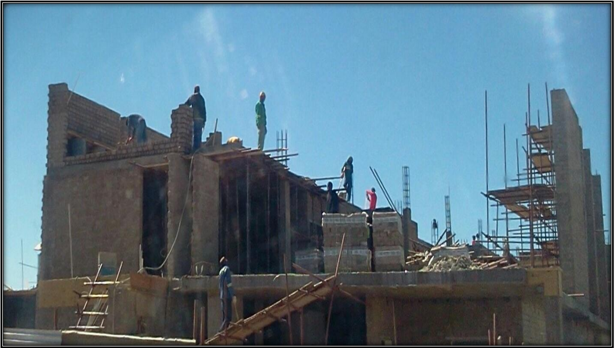
Figure 5.1 Picture taken from construction sites depicting workers not wearing full PPE
