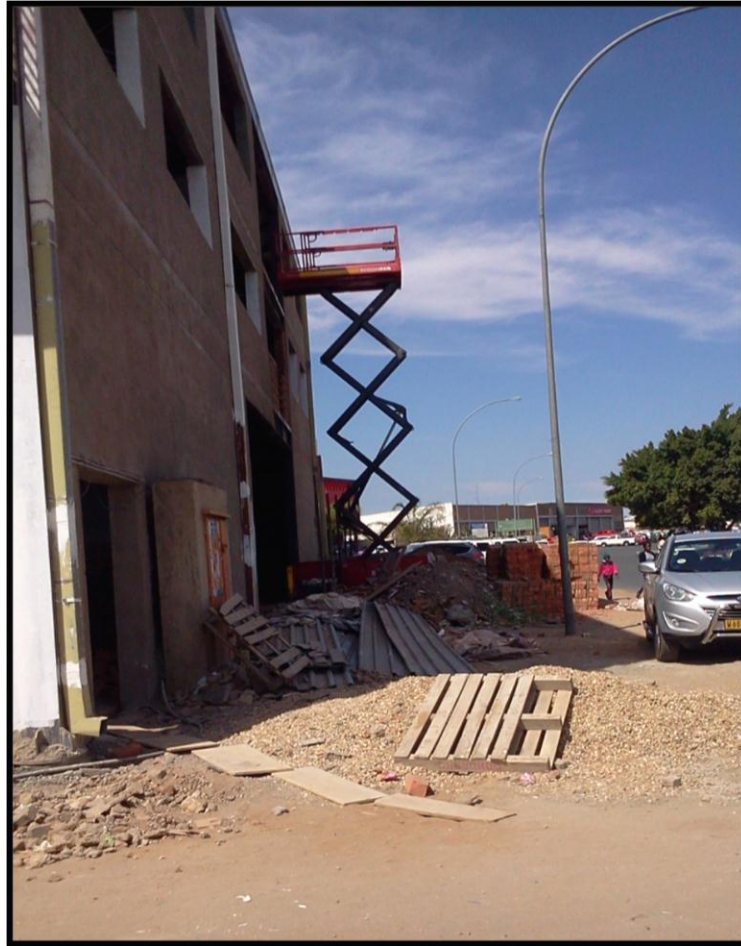
Figure 5.8 Construction site showing a lack of people or transport movement control measures
