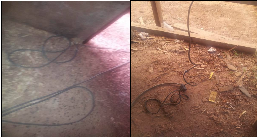
Figure 5.16 Photographs showing unsafe electrical connection and trailing electrical wires exposing workers to high risks of electrical shock
