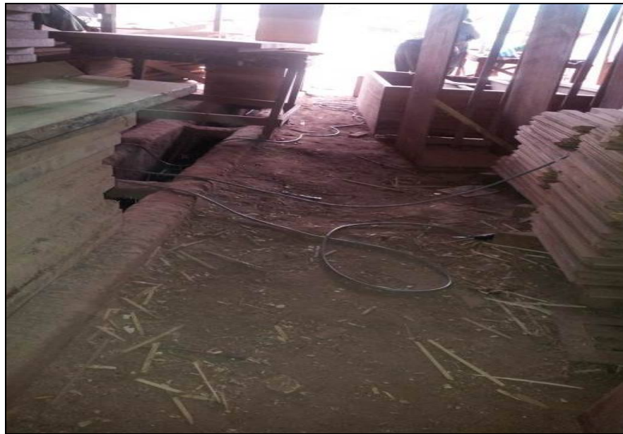
Figure 5.8 A photograph depicting electrical cables and packed wood obstructing the narrow walkways that can cause workers to stumble and fall resulting in serious injury
