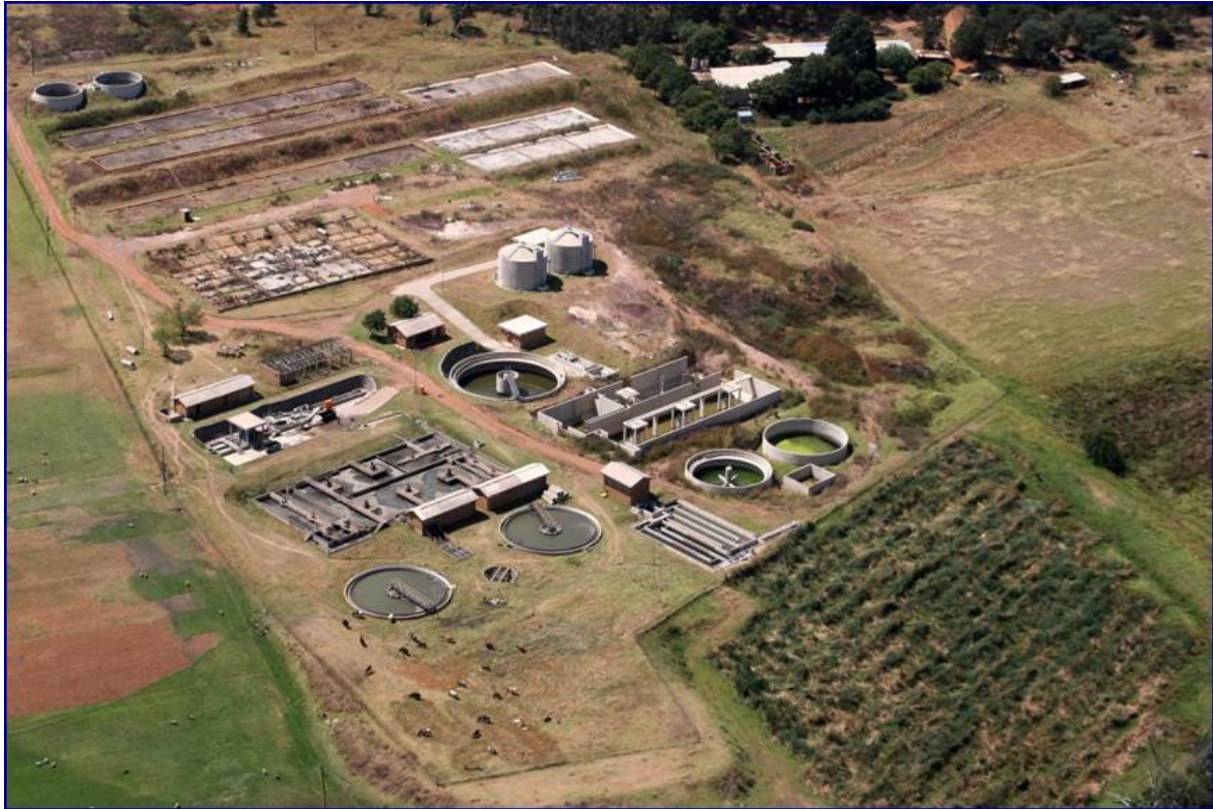
Fig 3.2: Sewage processing plant in the eMalahleni (Witbank) municipality not fully functional and discharging raw sewage in the upper catchment of the Olifants River (picture: Johan Eksteen)
