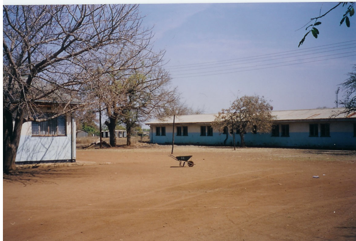
IMAGE 4-3 A view of the school showing some of the classrooms
