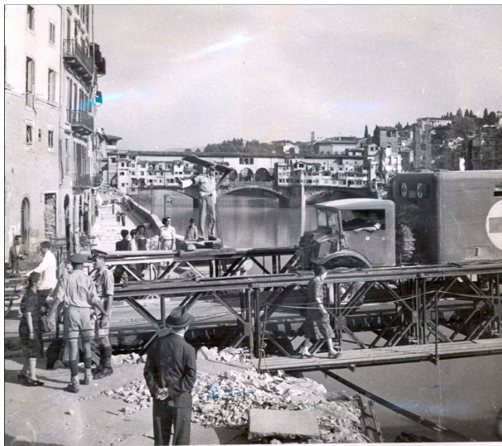
FIGURE 8: Bailey bridge in Florence, Ponte Vecchio in background. FROM: Ditsong National Museum of Military History.
