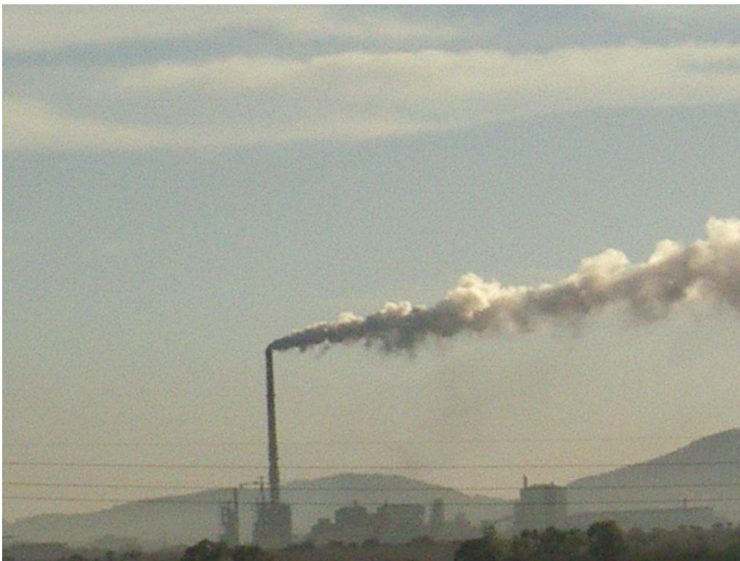
Figure 4.13: Example of Smelter emissions (black part of cloud is particulate emissions) (North West Ecoforum, 2002).
