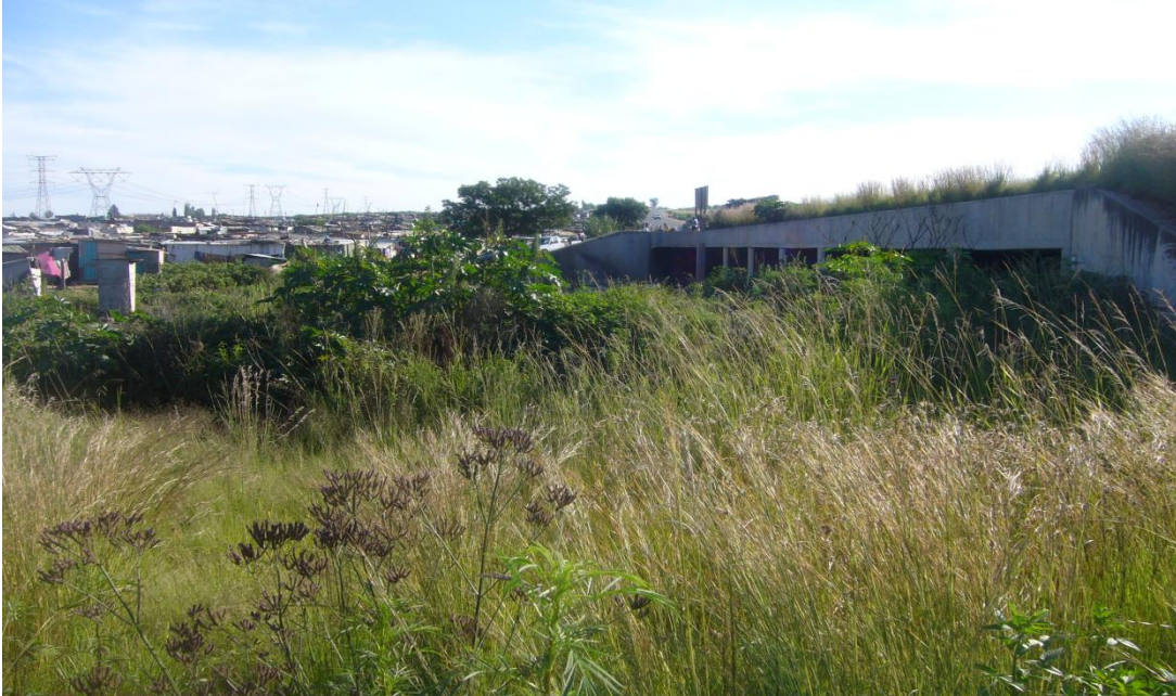
Picture 1.1: Depiction of Ivory Park informal settlement situated next to multiple storm water pipes and heavy electric cables
