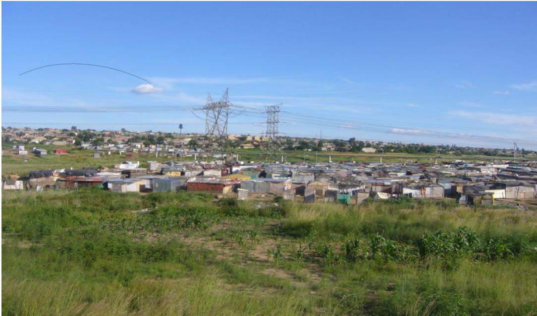
Picture 2.2: Ivory Park informal settlement depicting shacks, high voltage electric cables and sewerage pipe running over some shacks
