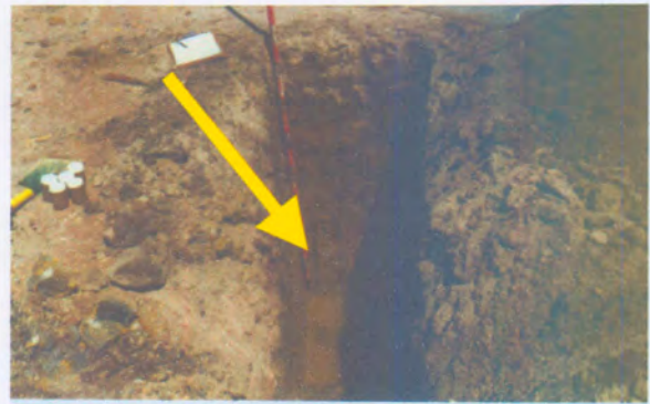
FIG. E.10 - Seepage in test pit C/2. A sample was taken for chemical analysis.
