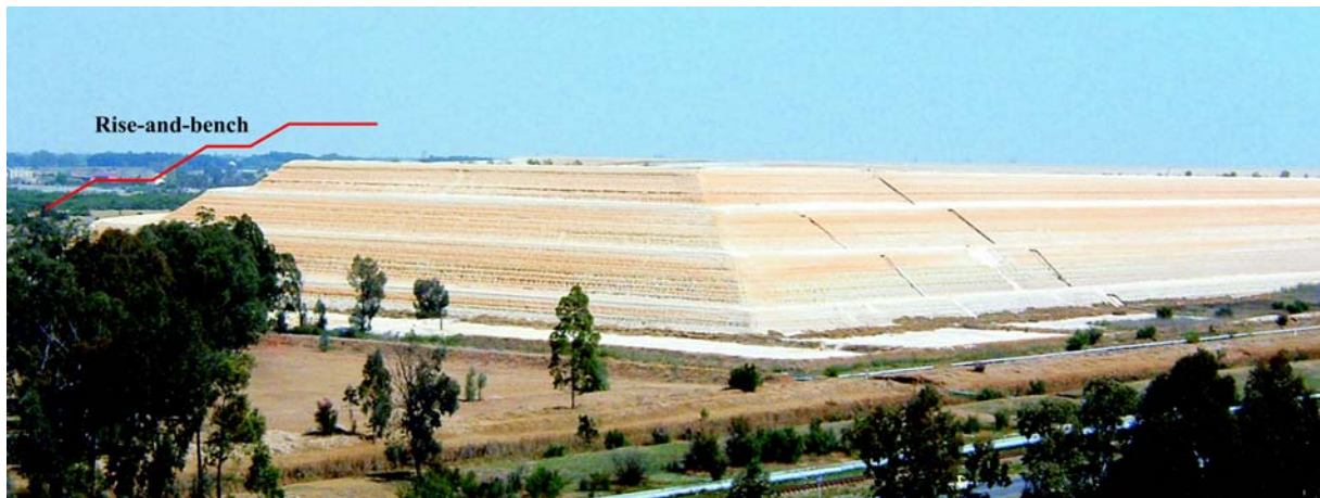
Figure 74: Typical side slope profile of an upstream constructed ring-dyke gold tailings impoundment.
