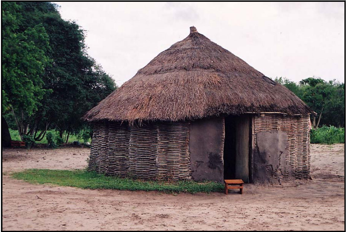
Figure 8: A round storage house. The walls of the house are made of a wooden lattice stacked between larger supporting poles and partly covered in mud. The roof is thatched. The storage house is no different from other constructions except that it usually has no windows. At 12 years since construction, this particular house was among the oldest wooden structures sampled by Gaugris (2004). Photo by J. Gaugris: Manqakulane community, northern Maputaland, KwaZulu-Natal, South Africa, 2002.
