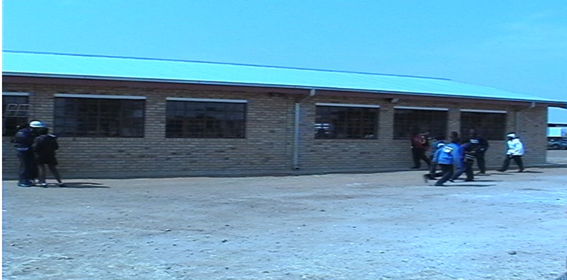
Self produced photograph (28/03/2003) 3 (e): shows the new additional administration block built from the infrastructure capital project.
