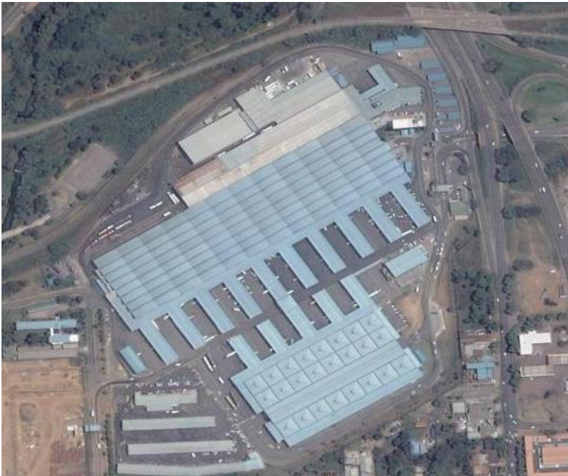
Image 8.63: Aerial view of Pretoria market Source: Google Maps (2015b)
