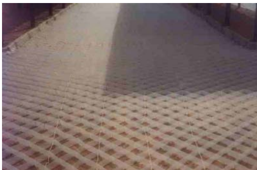
a) Unfilled geocell mattress.
