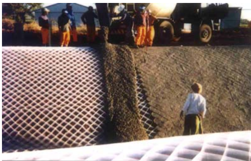
e) Geocell channel lining being filled with concrete.
