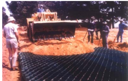
b) Mattress being filled with soil.
