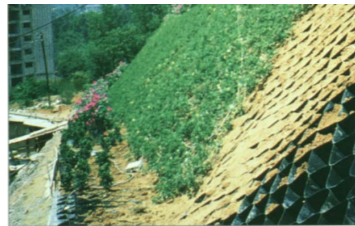
f) Geocell retaining structure.
