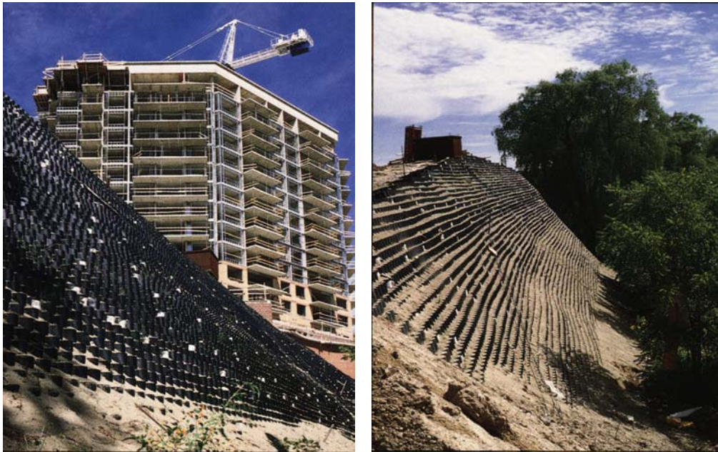
Figure 2.3 Geocell applications in retaining structures (with courtesy from Geoweb cellular confinement systems).
