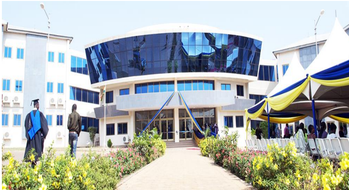
Picture 3-2: The front view of the Administration Block for the sheep institution
