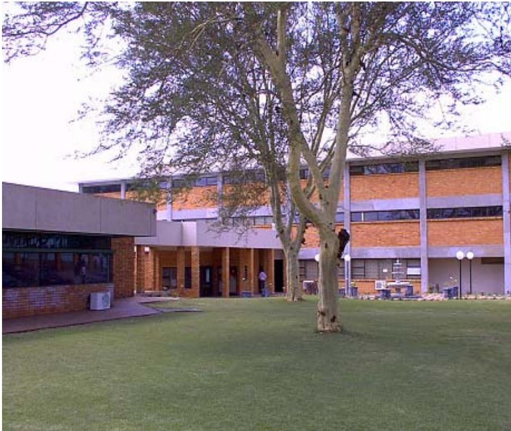
Photo 2: Pretoria West College of Engineering
