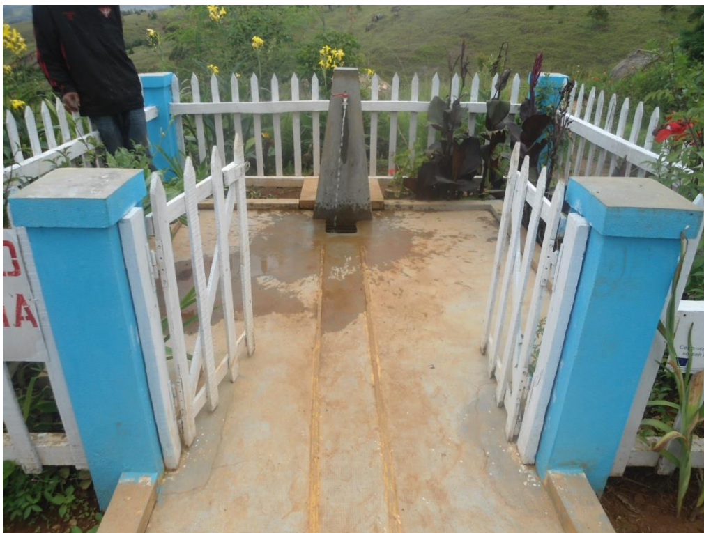
Figure 15. TYPE DE BORNE FONTAINE IMPLANTE A SOANIADANANA
