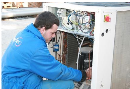
Figure 1.4 Maintenance et services
