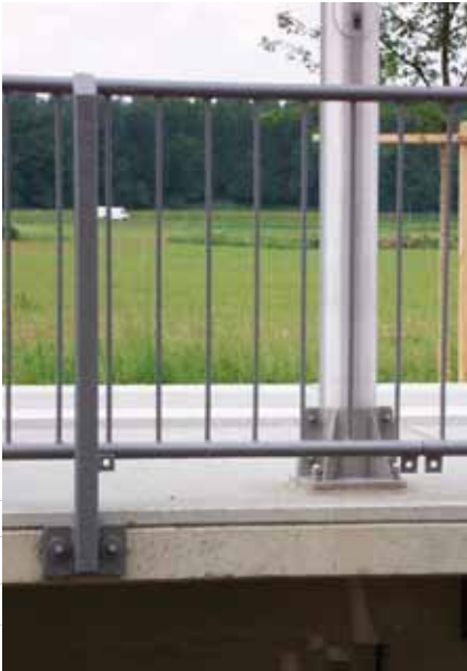
Railing and lamp post anchoring
