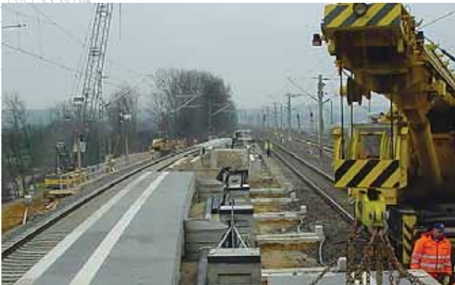
Cologne Weiden-West with conventional centre core backfilling - type 3a
