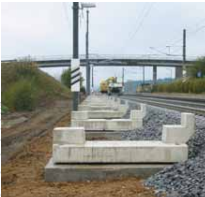
Foundations for types 1a and b
