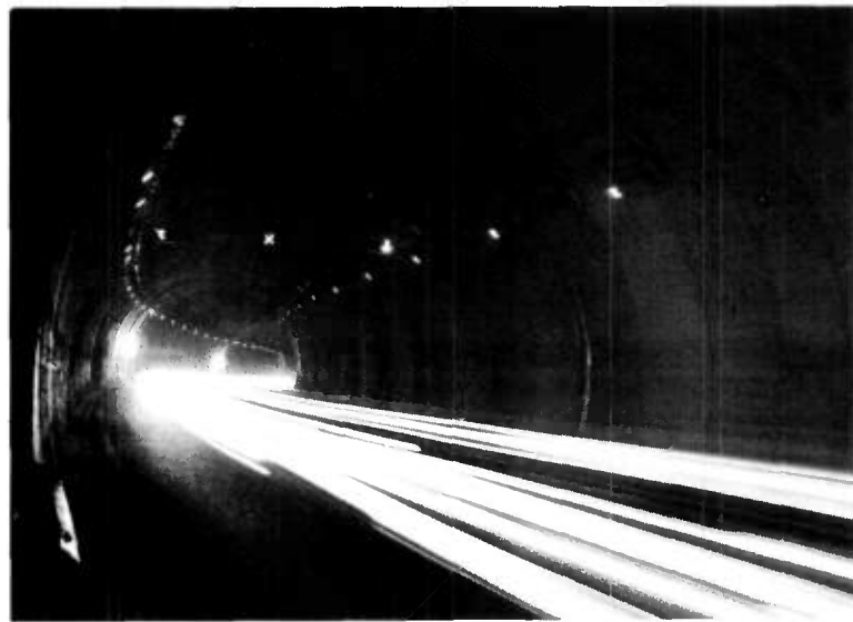
Figure 38. Autoroute A. 8. - Tunnel de la Baume.
