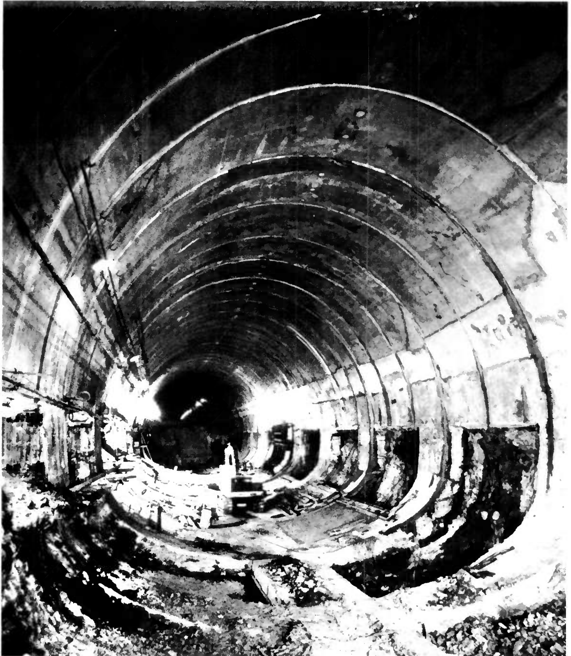
Figure 12. Tunnel André Malraux (Cimiez) - Nice.
