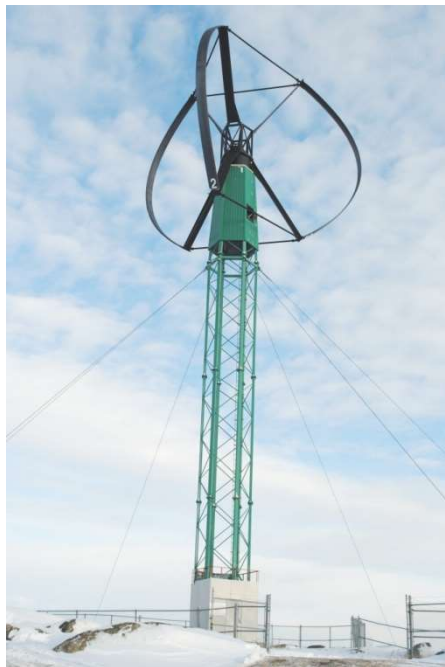
Figure I-2 Overview of the Cap d'Ours wind turbine.
