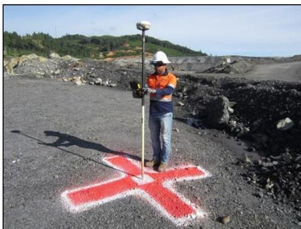
Figure 2.8 Marquage de GCP (<https://support.dronedeploy.com/docs/working-gcp-step-by-step>)
