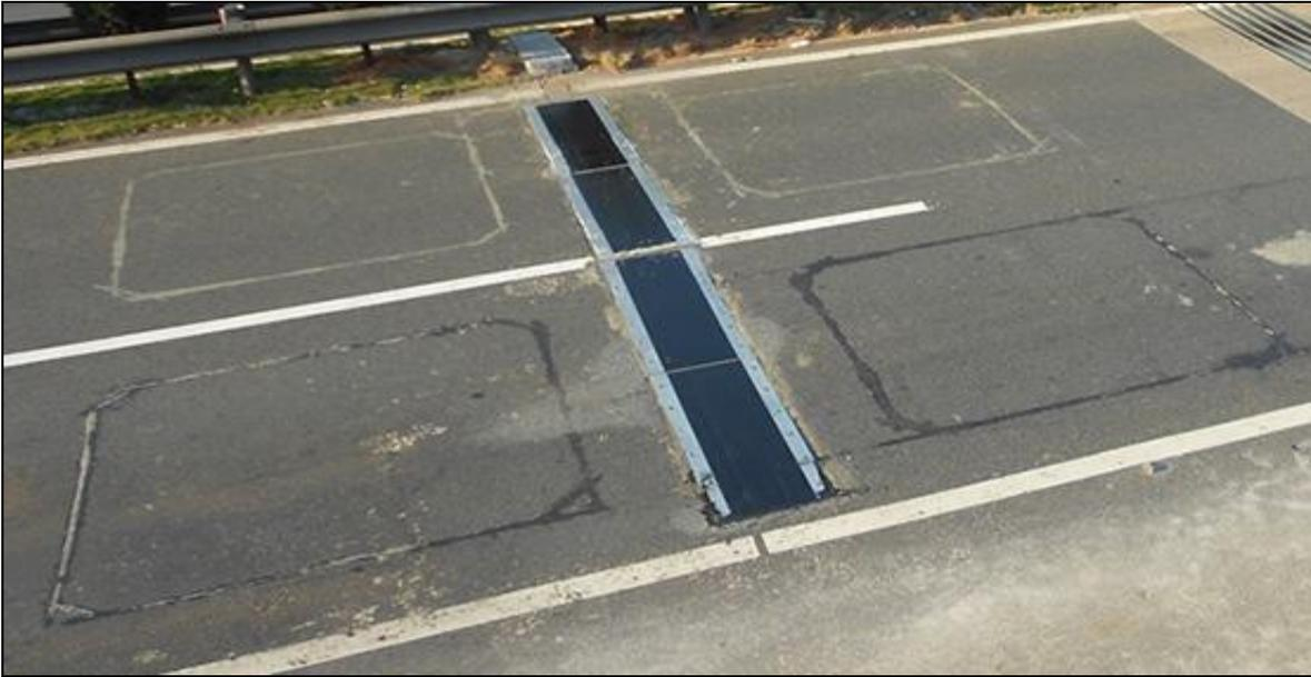
Figure 3.21 Plaques de pliage (<https://www.viscoindia.com/bending-plate-medium-speed-weigh-in-motion-mswim.aspx>, 2018)
