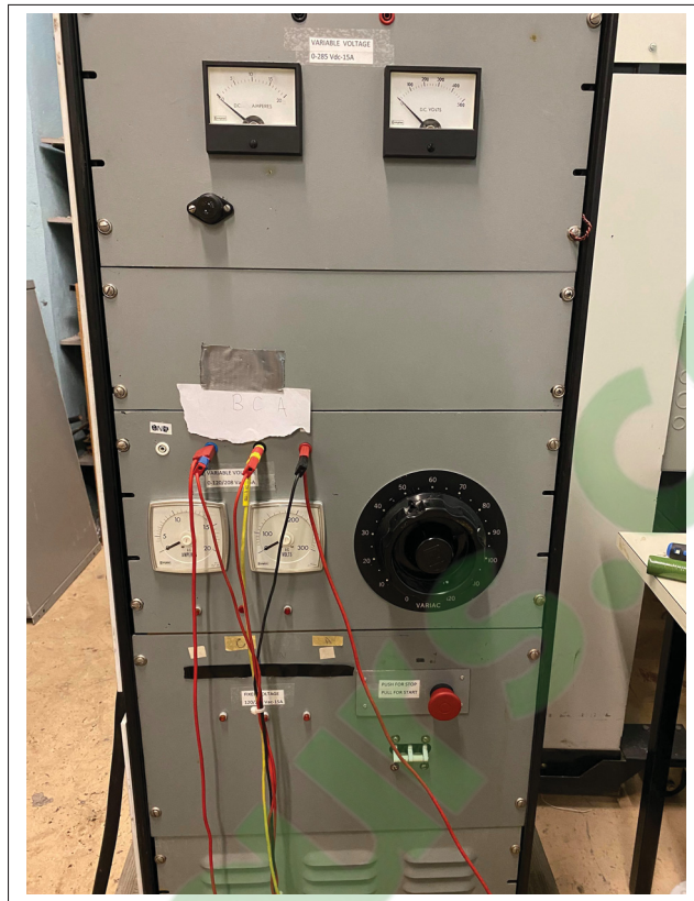
Figure 6.3 Excitation transformer used during experiments
