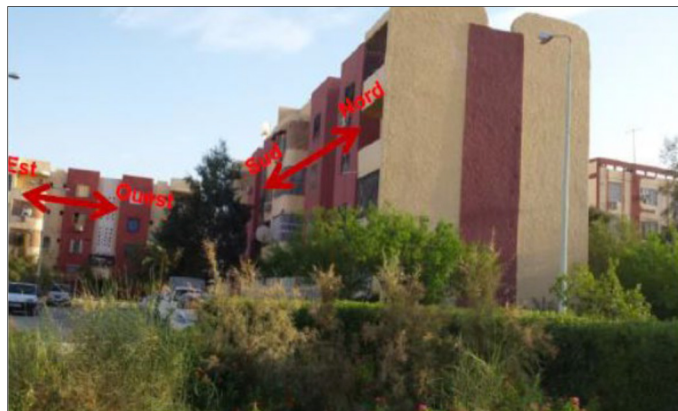
Figure 4-3: Residential buildings built in the 1980s
