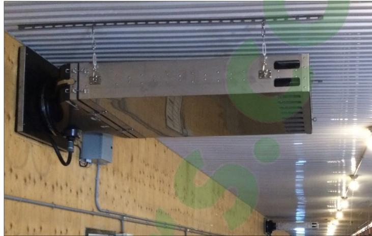
Figure 2.3 Counter-flow air-to-air HX unit installed in a broiler house
