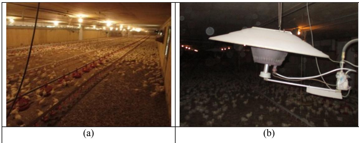
Figure 2.2 a) View of the broiler house studied b) A typical radiant propane heater
