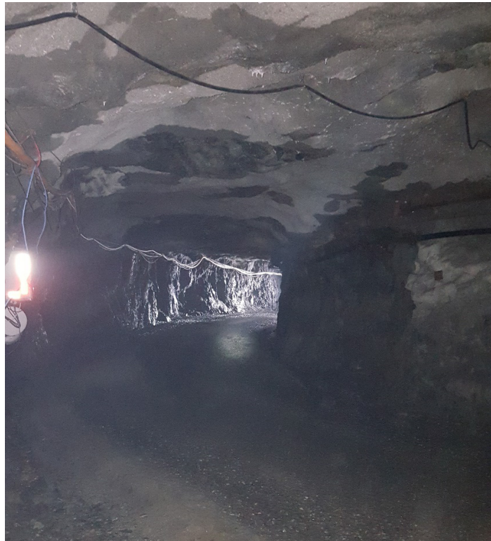
Figure 41: Photography of the mine gallery.
