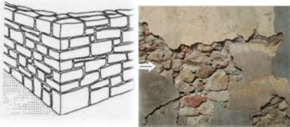
Figure 2.22 :mur en moelons
