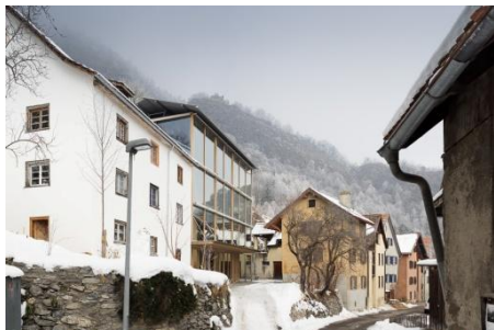
Figure 48 – Atelier P. Zumthor, Dorfasse, 2016.
